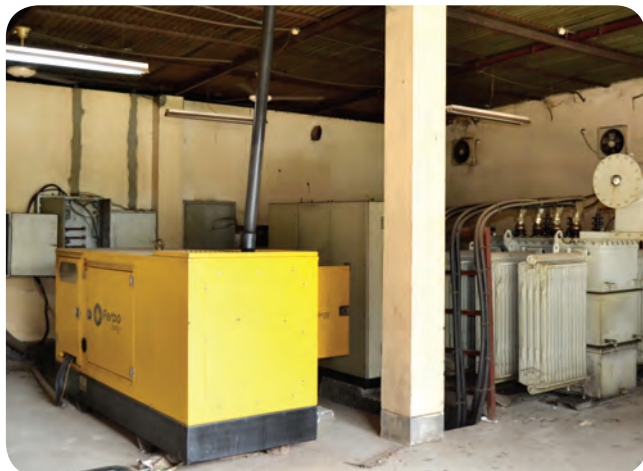
Installation of electricity sub-station at PSC
