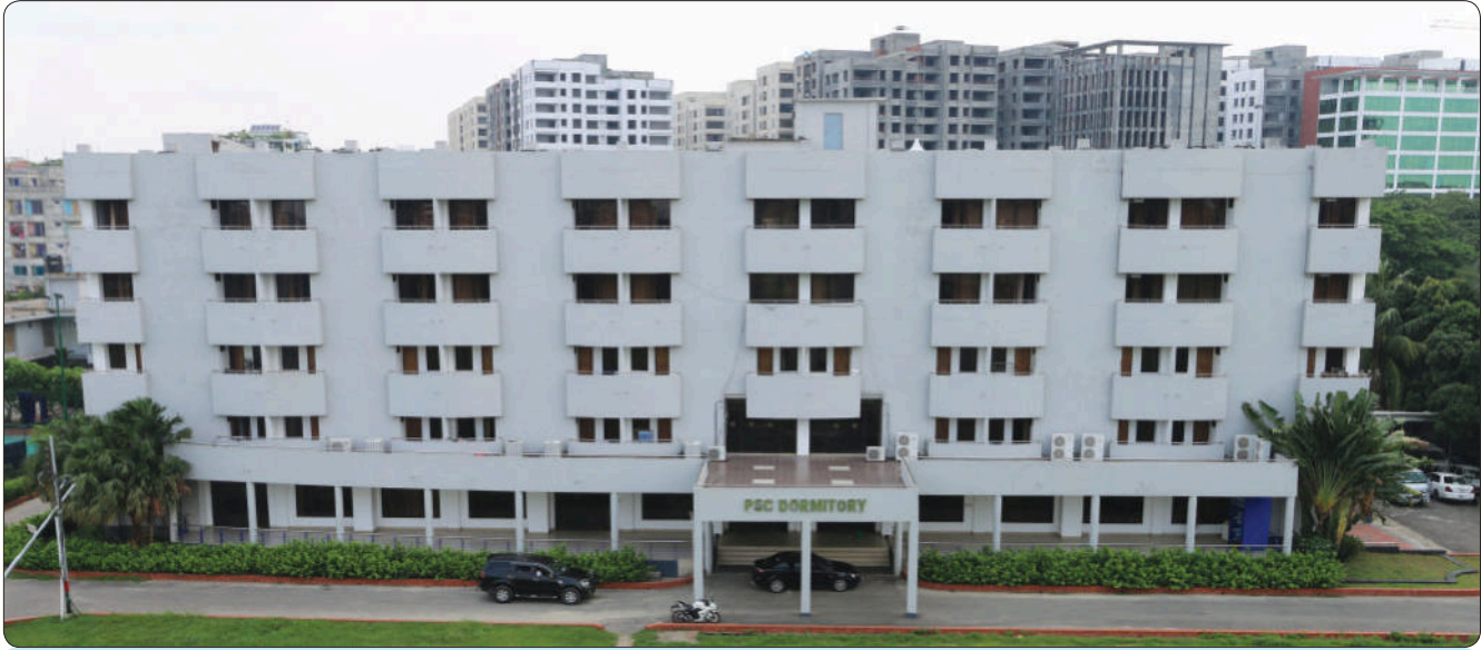
Five-storied Dormitory at PSC
