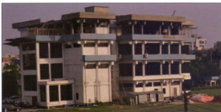
Progress of vertical extension of PSC academic building
